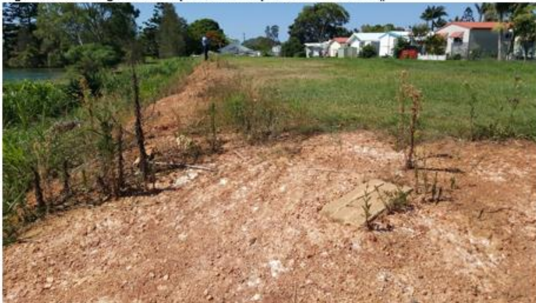
Figure-6: Building materials present in exposed batter of fill.
